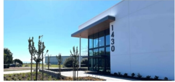
GMP manufacturing, product testing, and storage (~92,000 sf) - Alameda, CA
